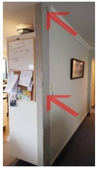
Cracking evident to the ceiling plaster join here. Not of a structural concern. Remedial attention required, Cosmetic upgrade required.
