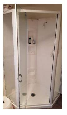
The mid section of the shower liner is not sealed back tight to the wall here. The shower appears watertight however in time be aware this liner may require re-glueing and sealing.
