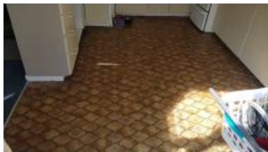
Damaged vinyl evident
