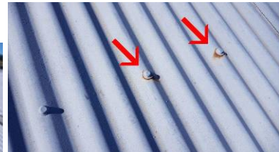
Rust evident to roof lead head nails
