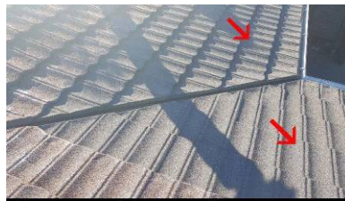
Newer roof over patio areas at base
