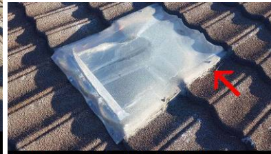
Surface sealed skylight area
