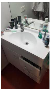
Plumbing:Flexi hose installed here. No plumbing running<br/>in the wall cavity was viewed, the plumbing<br/>product is unknown unless viewed in the<br/>subfloor or ceiling space and this will be noted<br/>on in their respective areas of the report.<br/>The waste pipe in this area is modern PVC.Vanity Unit Top:Enamel, Reasonable Condition.Vanity Unit Other:Doors, Good Condition, Drawers, Good Condition.Vanity Unit Taps:Single water mixer, Reasonable water pressure.
